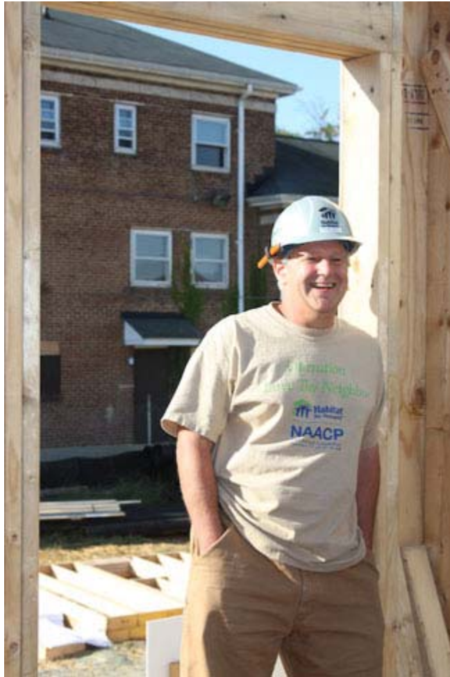
House leader Steve Buck, who serves on the board of directors of Habitat for Humanity of the Chesapeake, said it is good to be working on a Carter project in his home territory. ©Habitat For Humanity/Angel Pachkowski
