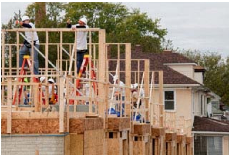
Volunteers work on the 10 new houses being built in Annapolis, Maryland's Clay Street neighborhood on Day Two of the 2010 Jimmy & Rosalynn Carter Work Project. ©Habitat for Humanity/Steffan Hacker
